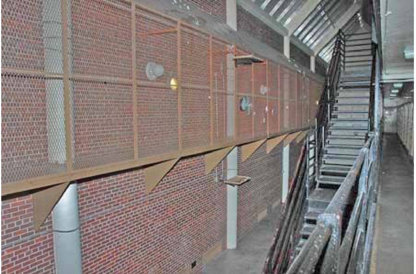
View of protected walkway from cells
