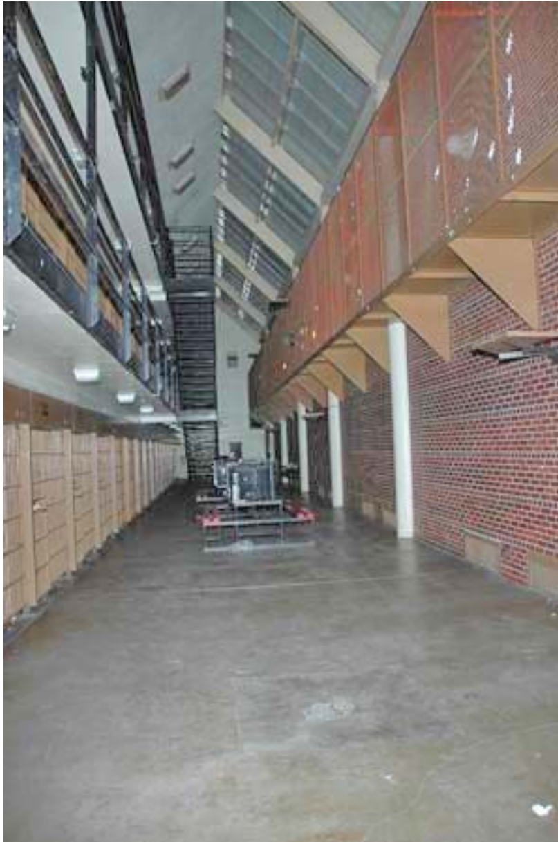
Cells with protected walkway
