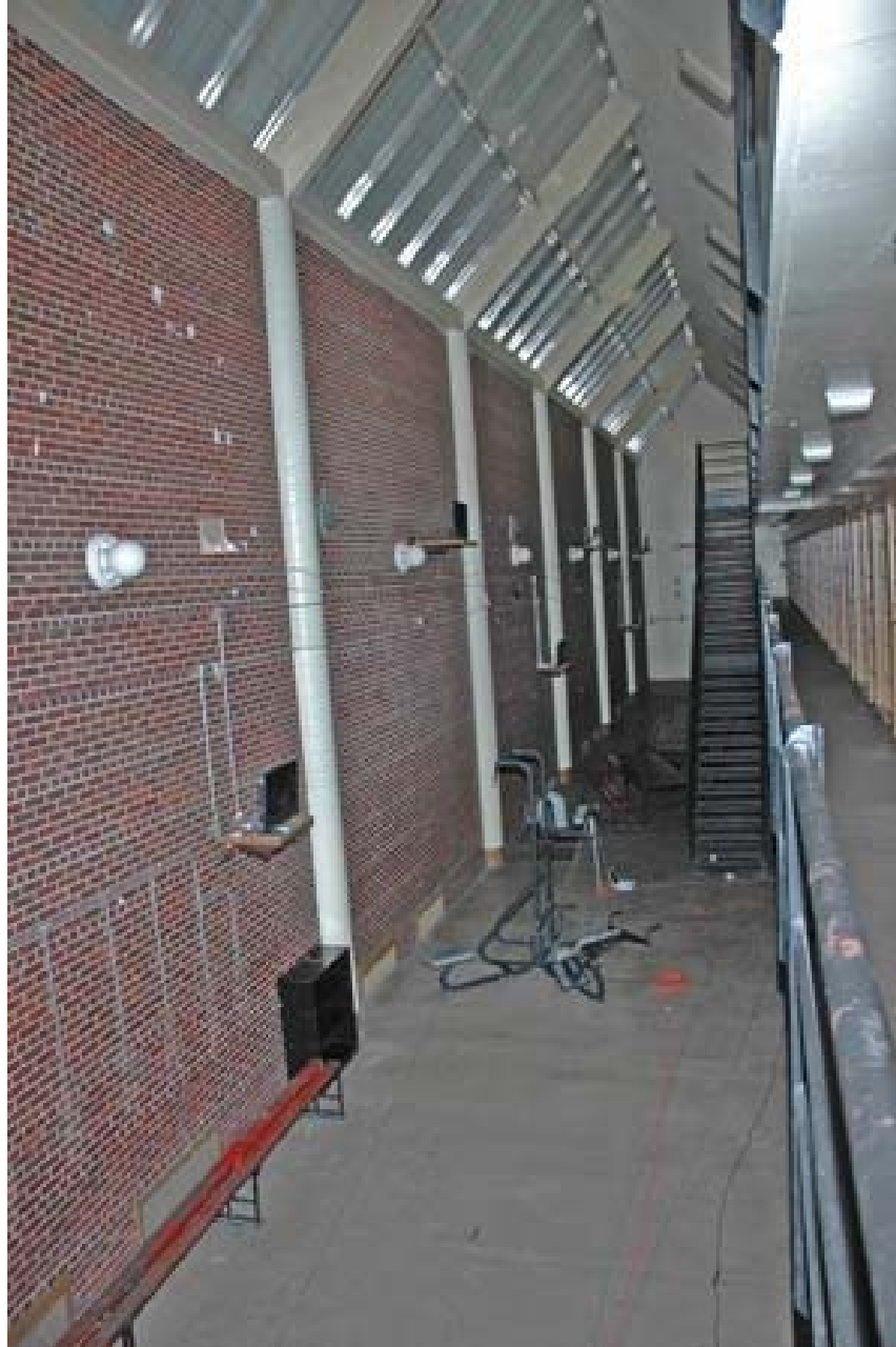
View of the third tier on first night
