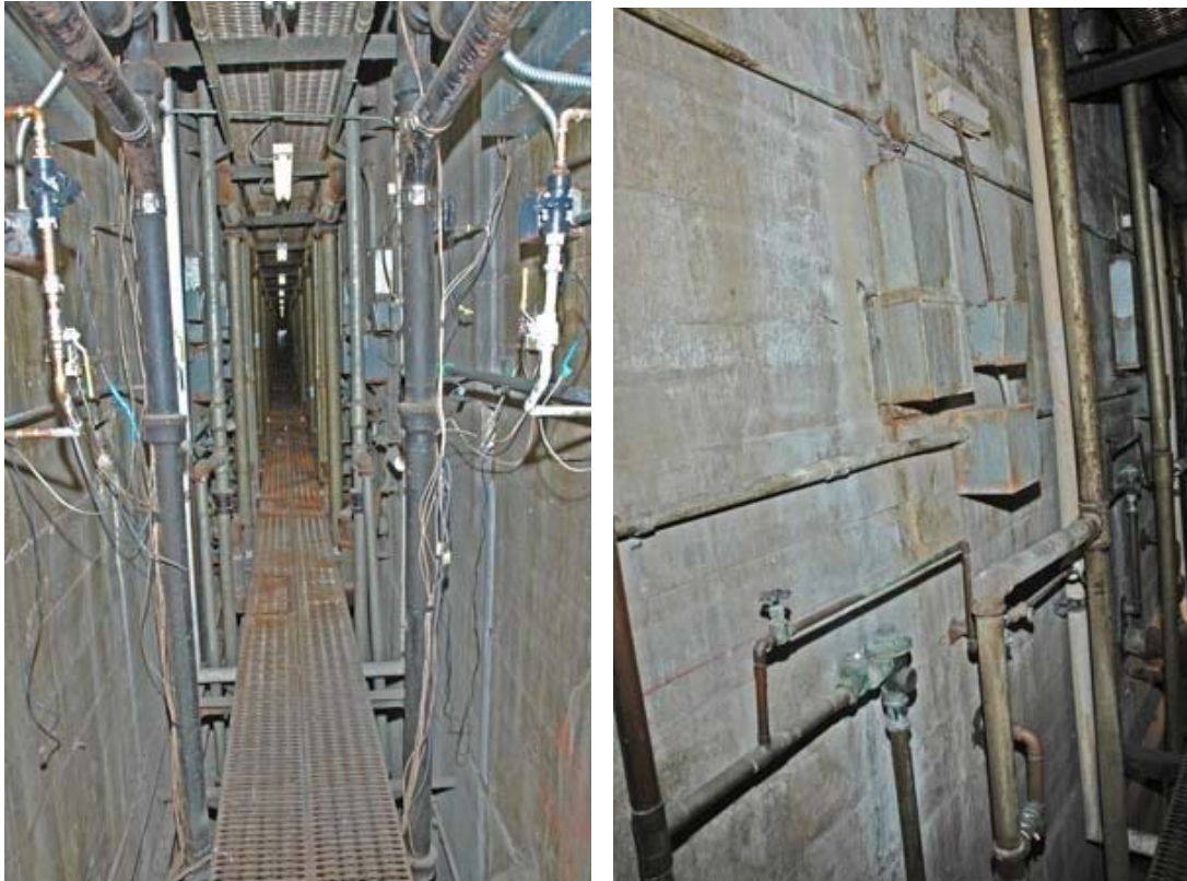
The Pipe chase area between the cell blocks
