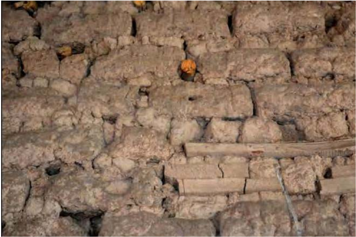
Example of original adobe wall
