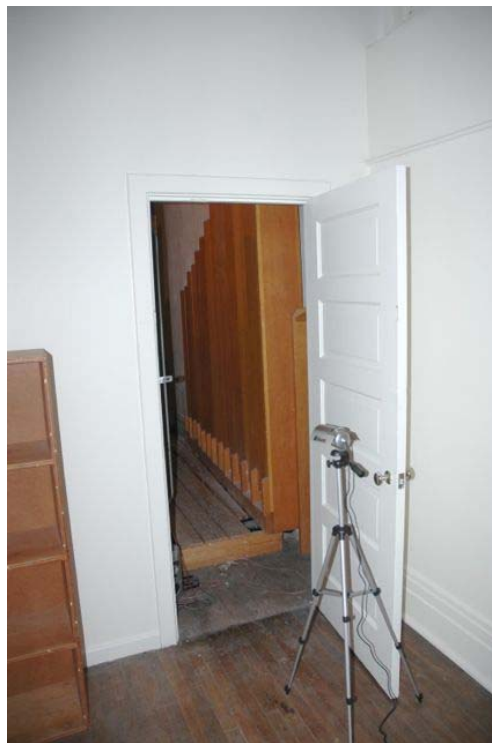
Entrance to pipe room
