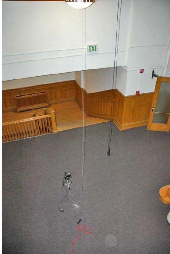
View from tower entrance to lower floor
