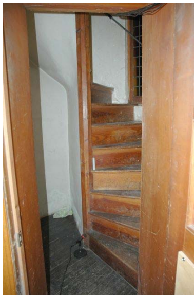
Stairs leading to tower room
