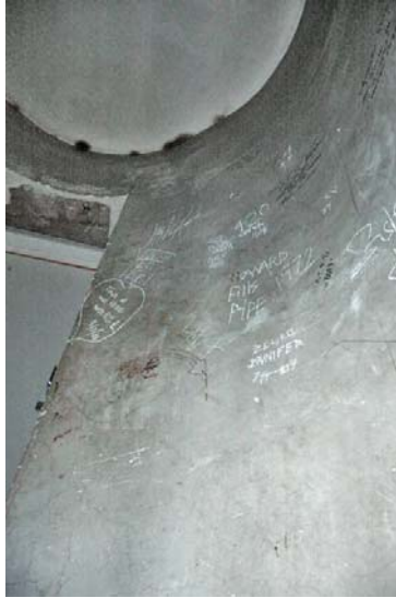
Wall in tower
