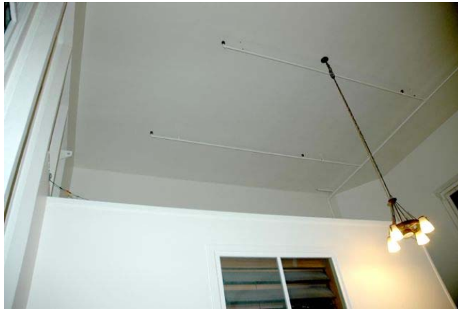
Ceiling of the tower room
