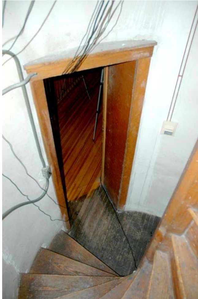
View down to tower room entrance
