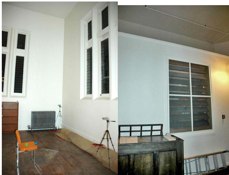
The tower room
