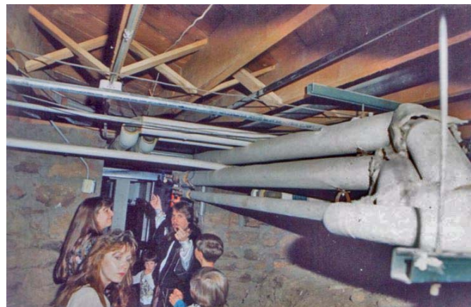
Inside the "Tunnel"
