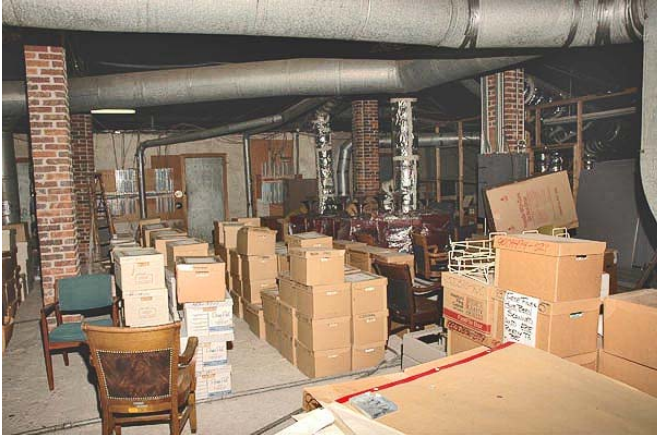
Storage area in attic
