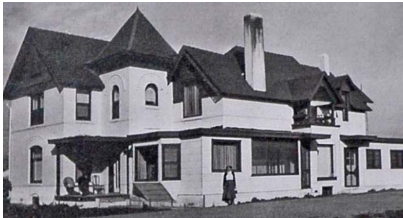
One of the final remodels of the house
